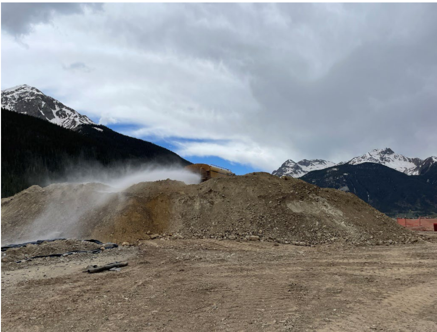
Water truck sprays down a pile of material for dust suppression.
