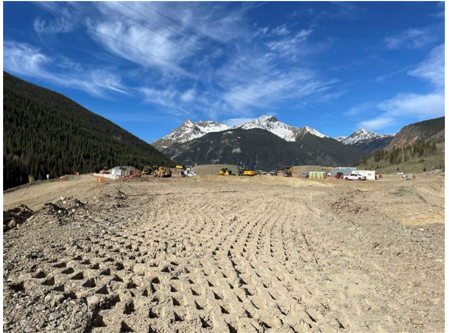
Compacted material lays the foundation for the facility
