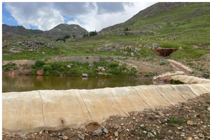
A berm constructed to manage surface water near the Sunbank Group Mine
