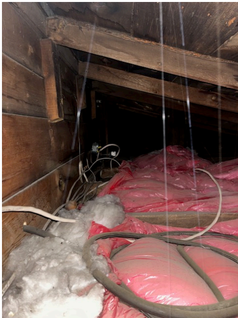
Under structured roof framing Random wiring and open junction boxes Fire Hazards
