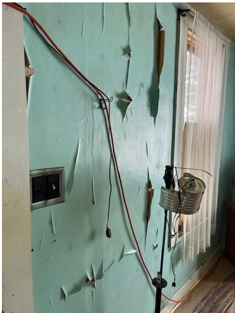
Current home wiring is random extension cords running where needed. Existing Interior walls
